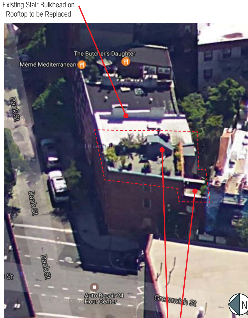
Aerial view of 769 Greenwich Street looking East along Bank Street
