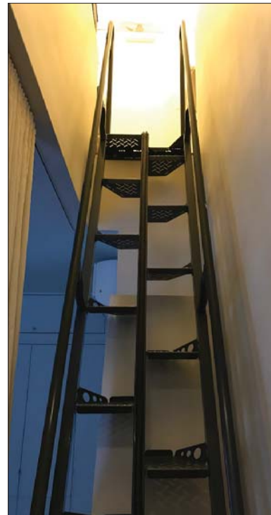
Photo of Existing Staircase to the Roof
