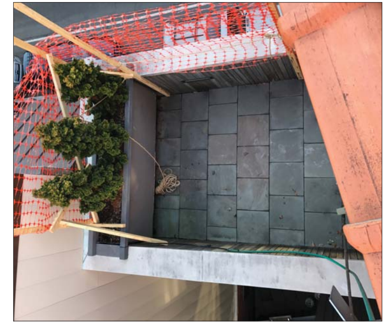
View of the Existing Third Floor Balcony from the Roofdeck
